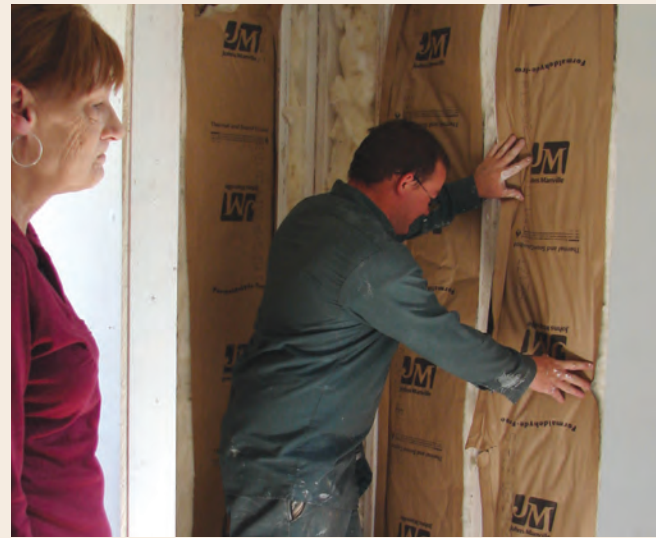
David Saveranzo of SERVPRO in Florence has been tearing everything out of Jackie Richardson's mobile home, spraying an odor-blocking agent, reinsulating the home, replacing sheet rock, etc. SERVPRO specializes in the cleanup and restoration of property after a fire, smoke or water damage situation.
